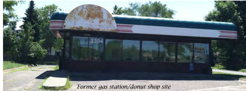
Former gas station/donut shop site
