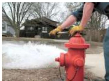
Public Works performs water main flushing after the snow has melted and the ground thaws; this year it is scheduled for the week of April 25, between the hours of 7:00 a.m. and 4:00 p.m. Flushing the water mains is done by opening the fire hydrants and letting the water flow at a high rate, which removes sand and sediment that has settled in the water main pipes since last flushing.
